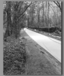
STABILIZED STONEDUST® TRUNKLINE TRAIL
