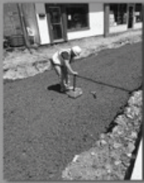
CU STRUCTURAL SOIL® EXETER, NH
